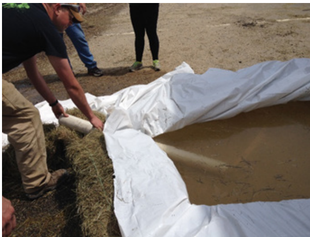
Rumford Fire – Building an underflow dam.
